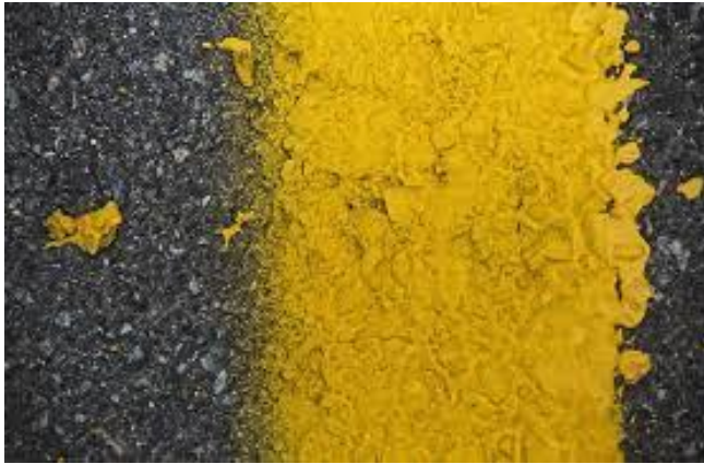
Figure 9 decaying paint
