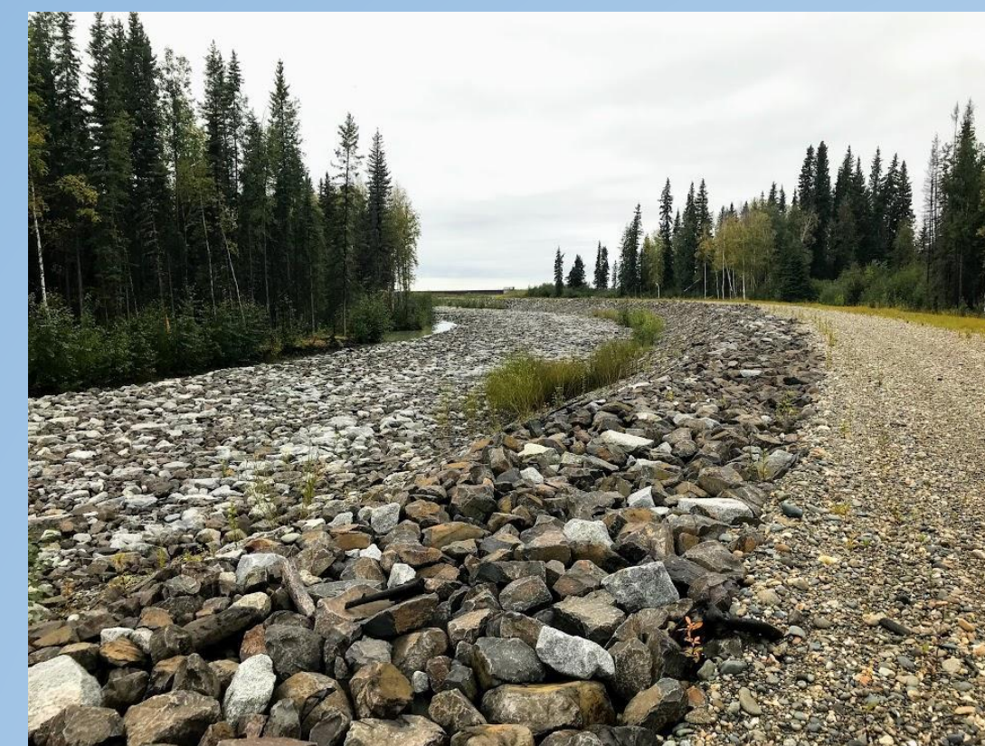
Tanana Crossing Levee Upriver from Bridge
