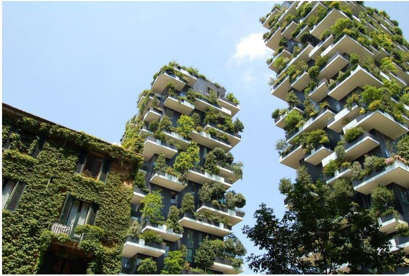
Picture 2 of Green Roof
