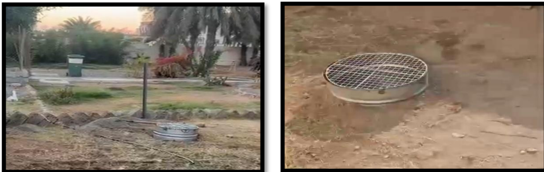
Picture (6): Preparing the Metal Tank and the Innovative Protection System
