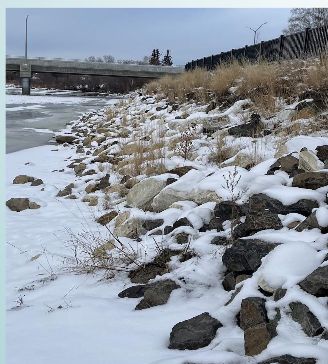
(Left) Bank reinforced with riprap
