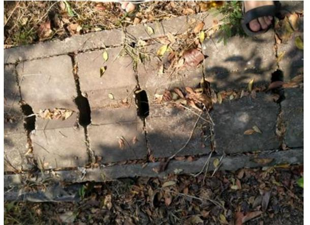
The drain pipe is closed. Figure
