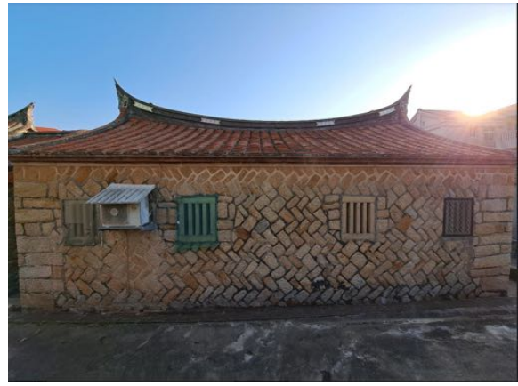
Picture of the back of the old house
