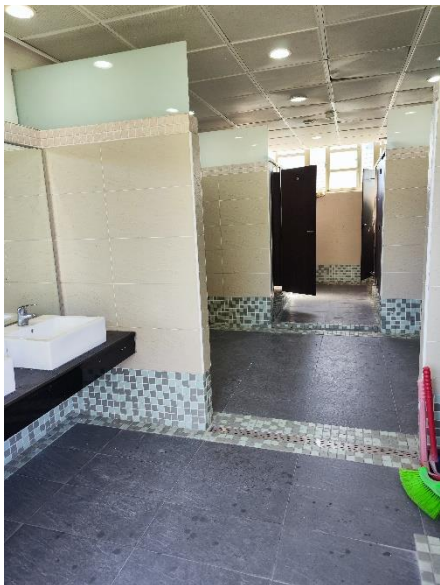
Toilet (wet floor)
