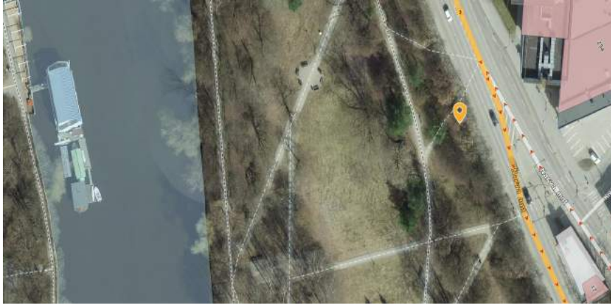
Figure 4. The location of the road site.
