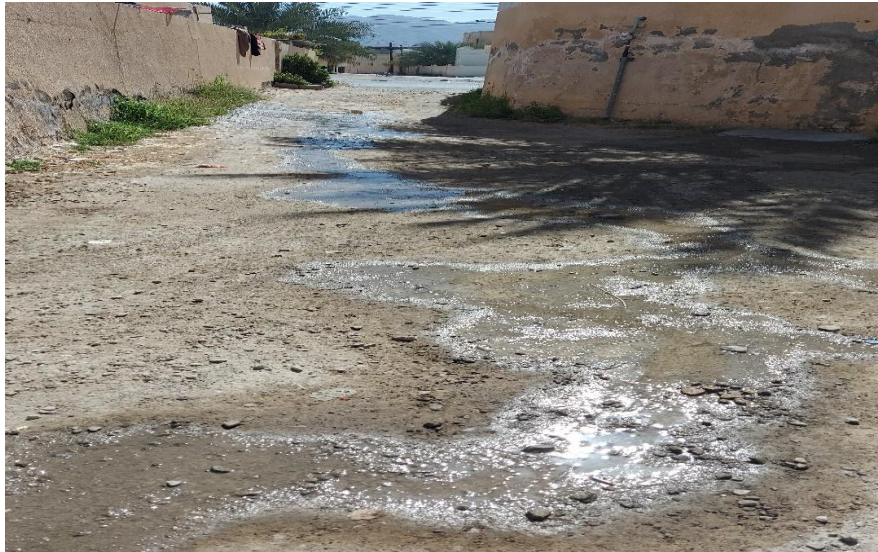
Photos (9) Grass growth on leak sites
