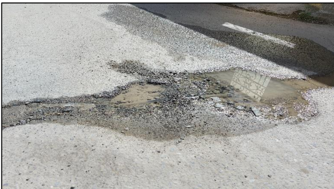
Photos (6) Some effects of leaking water
