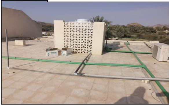
Starting the project by replacing iron castings with plastic seals
