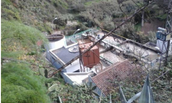
Picture 8: Water treatment plant La Bodeguilla.
