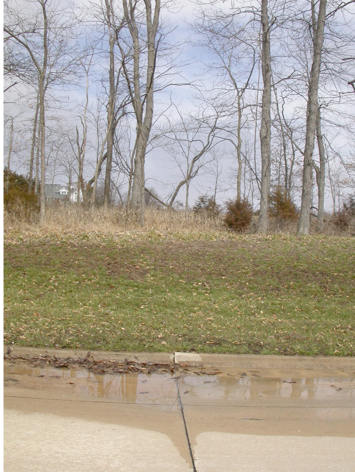
Figure 5. Puddle site, photographed in March, showing a gap in the curb and water seeping up through a crack in the road.
