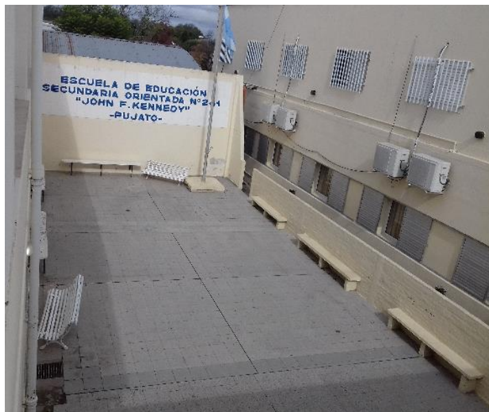
Figure 4: View of the site with the surface of the tiled floor
