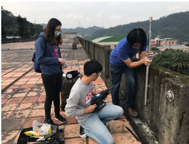
Davis weather station installation
