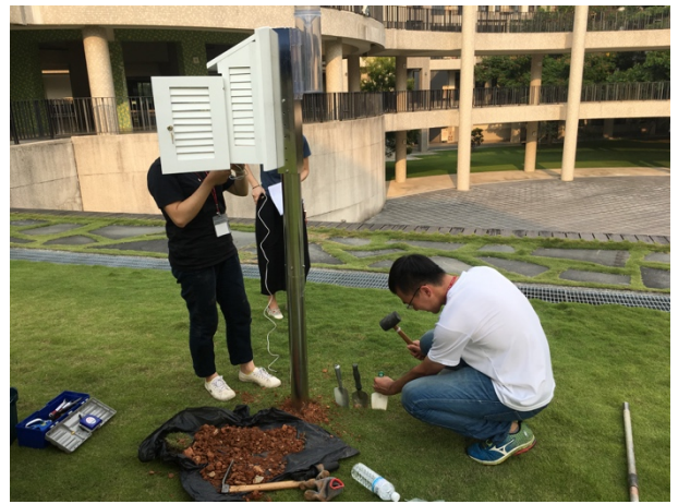
Building a shelter
