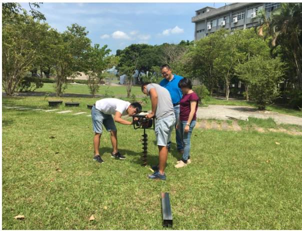
Atmosphere site installation
