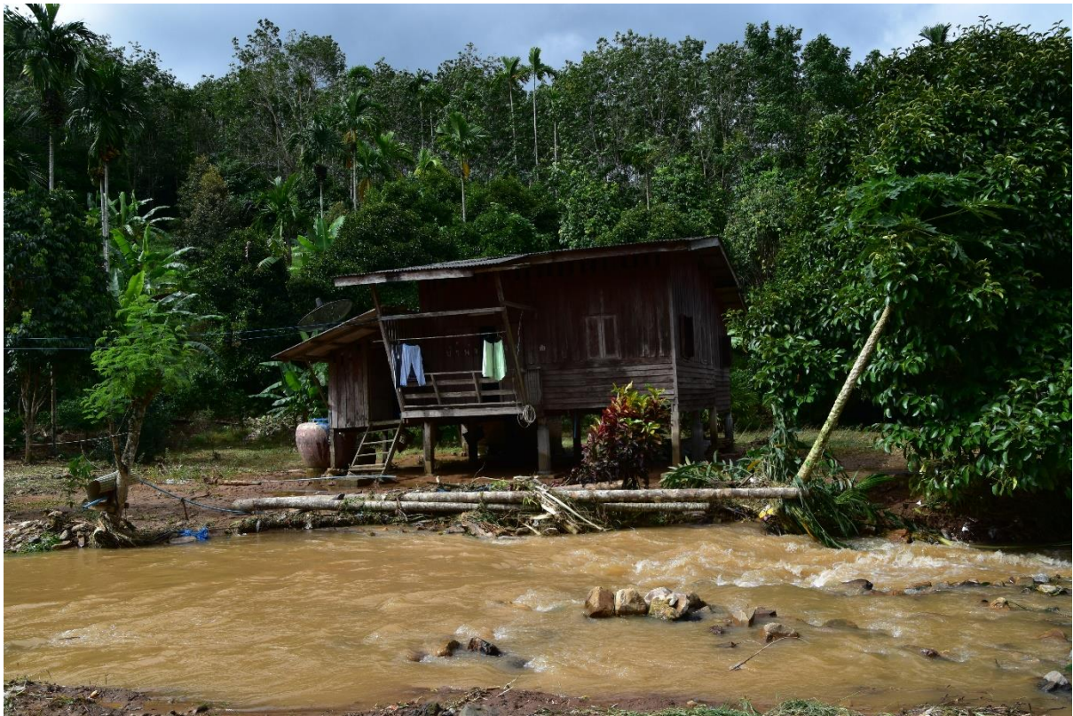
Traditional Thai houses with high floor level are not damaged during flooding.
