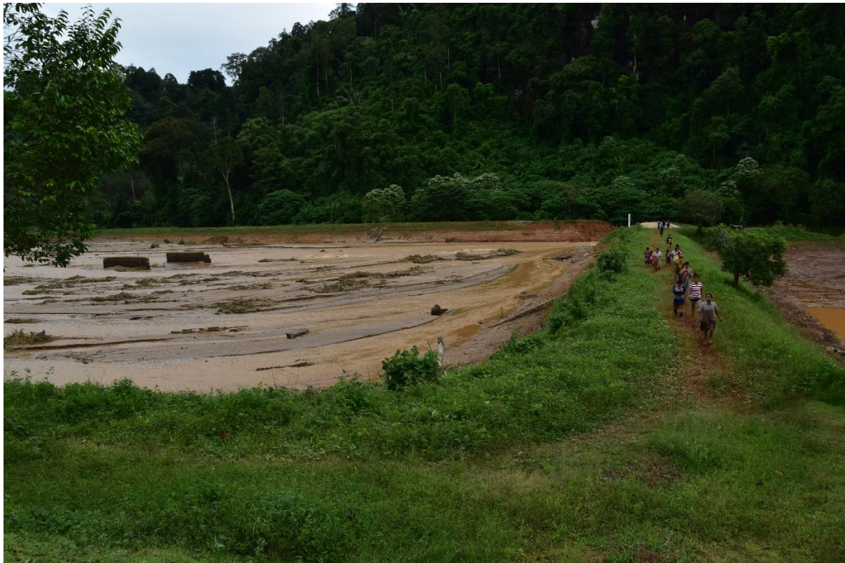
Figure 30 The reservoir was destroyed due to overflow of water.
